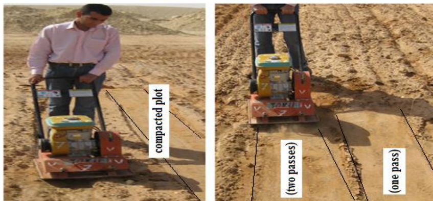
Fig. 4. Plate compactor was compacted soil during experiments
